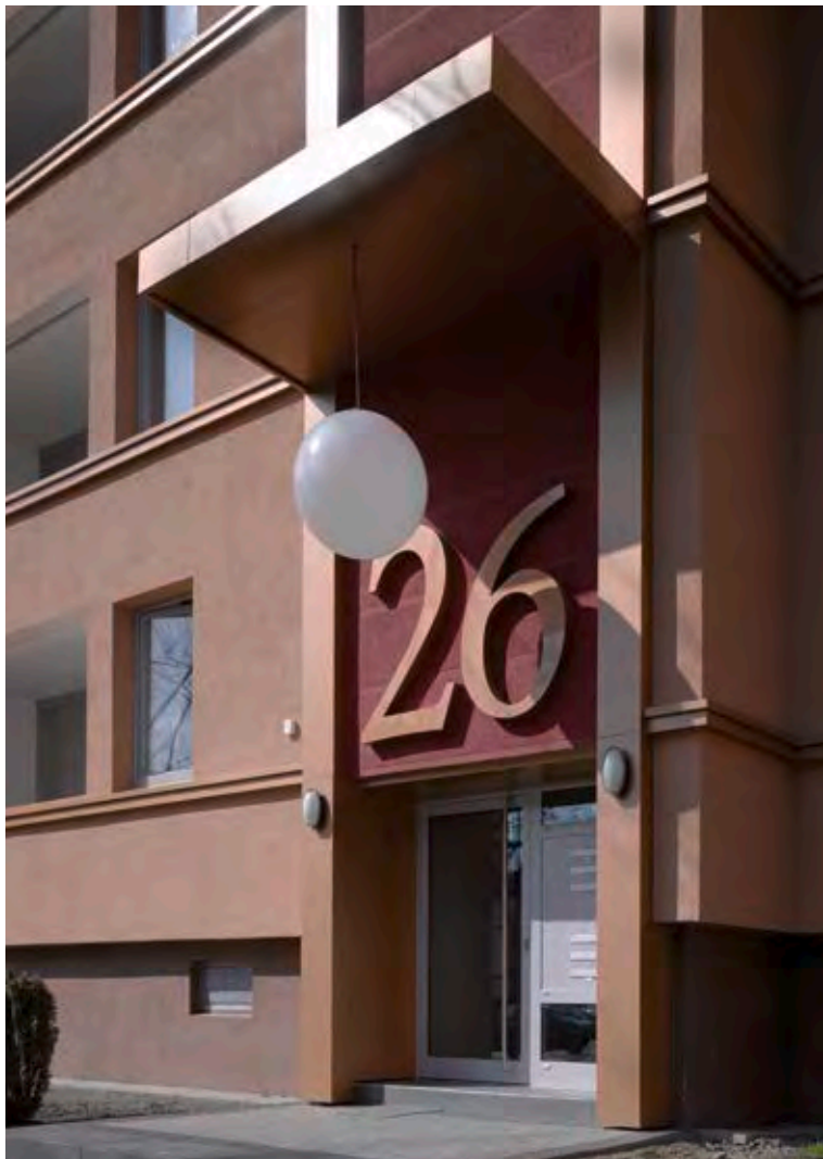
ALUCOBOND®-canopy with suspended luminaire; water-bearing level made of ALUCOBOND®
