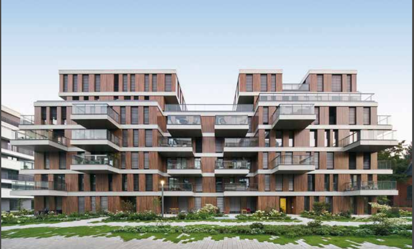
The Garden, Germany | Material: ALUCOBOND® PLUS legno European Walnut | Architect: Eike Becker_Architekten | Fabricator: BAM Deutschland AG | Installer: HMF Hübener + Möws Fassadentechnik GmbH | © Jens Willebrand
