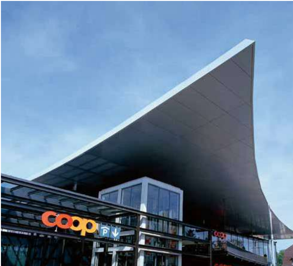
Stable – large, self-supporting roof with ALUCORE® cladding
